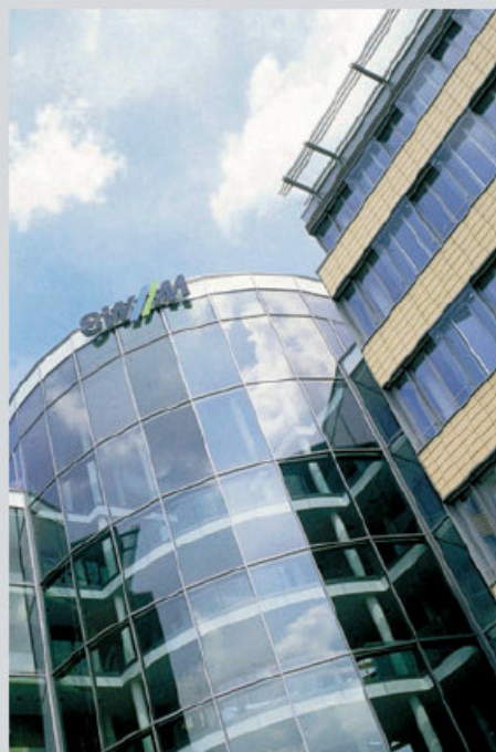
ECO at administrative building of Public Services, Munich
